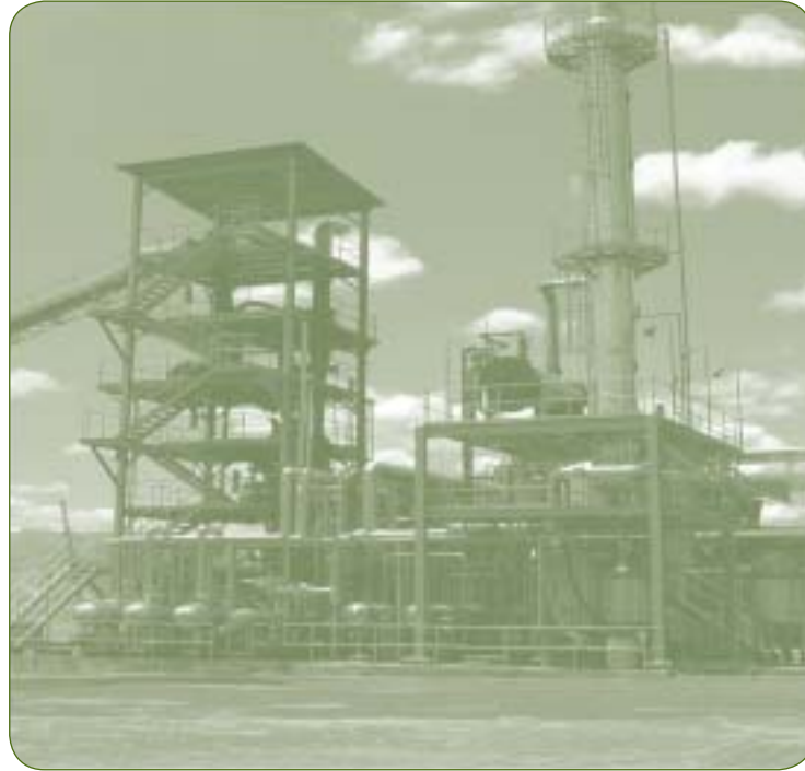
Dedini plant-pilot for producing bagasse-based ethanol.
